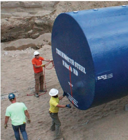
TrueNorth Steel underground storage tanks combine the strength of steel and the protection of fiberglass to create a durable tank that installs quickly. Our team partners with you to analyze the environmental risks at your site, and then offers you the appropriate internal and external protection recommendations. In addition, we are on-site during installation, to listen, learn and ensure our tanks are exceeding your expectations.
