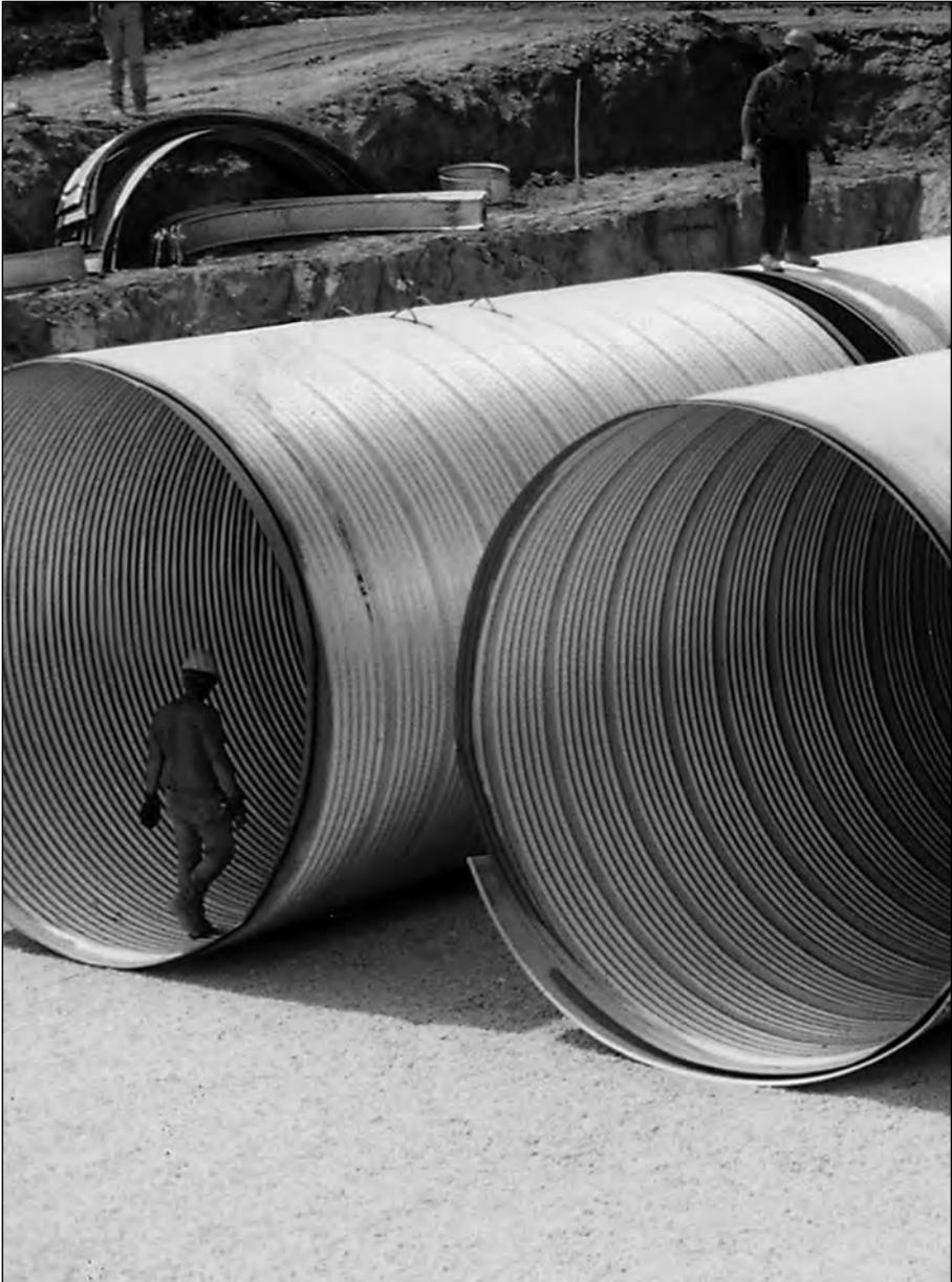
■ Typical CSP underground detention system.
