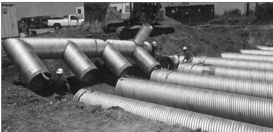
■ Typical CSP underground detention system.
