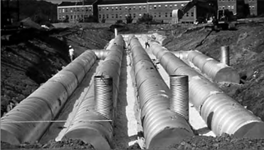
■ Typical CSP underground detention system.
