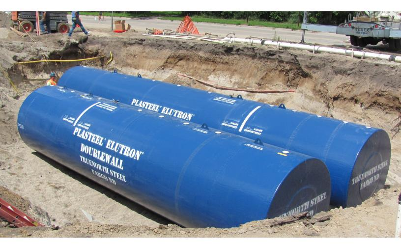
Each Elutron system is supplied with a factory-established interstitial vacuum. Prior to delivery, our team cleans and levels all the fittings and marks the center lines on each tank. These details save installers several hours of work normally spent on pre-installation testing and cleaning of non-metallic tanks.
