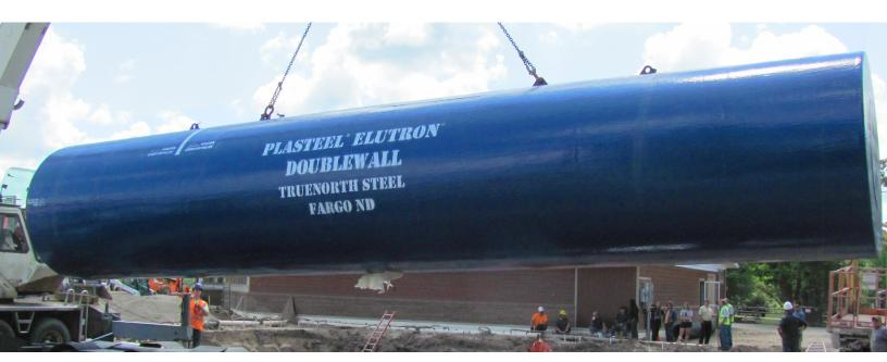
TrueNorth Steel Plasteel Elutron underground tanks can be supplied with pre-established interstitial vacuum and require a smaller excavation footprint and lower cost backfill materials than fiberglass reinforced plastic tanks.
