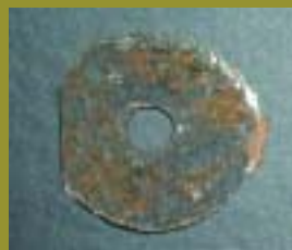
INVERT: SOIL SIDE
