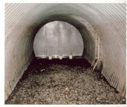
VERSATILITY IN FABRICATION. CSP can be readily fabricated into elbows, tees, manifolds, inlets and outlet control structures. This flexibility in design and system layout cannot be achieved with other materials. Also, plant fabrication means faster installation and lower job site costs.
