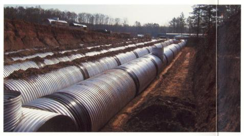
INFILTRATION. Where the proper soils are present, perforated CSP can be used as an infiltration system. This water quality practice duplicates undeveloped conditions by directing runoff back into the ground. CSP has the advantage of minimizing excavation, as compared to a conventional infiltration trench, and also allowing access into the system.
