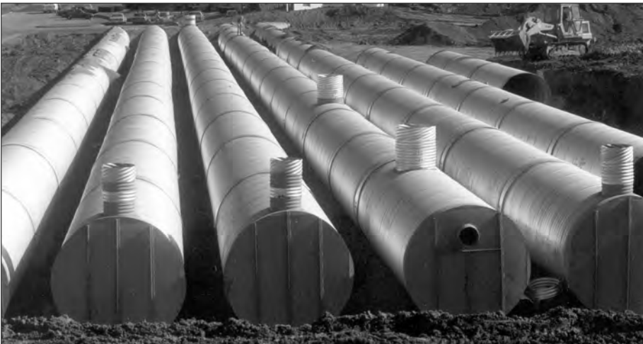
■ Shop attached CSP reinforced bulkheads.
