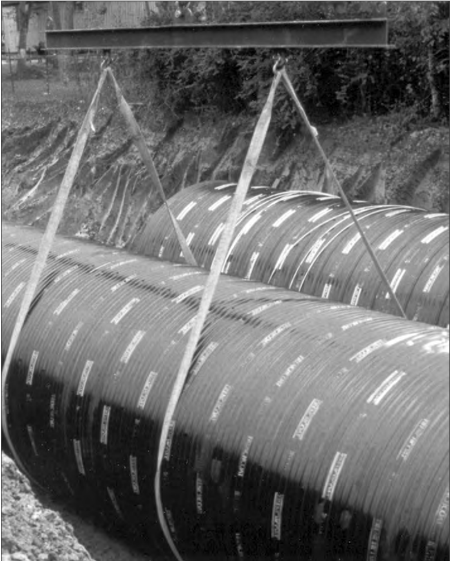
■ Installation of polymer coated CSP.
