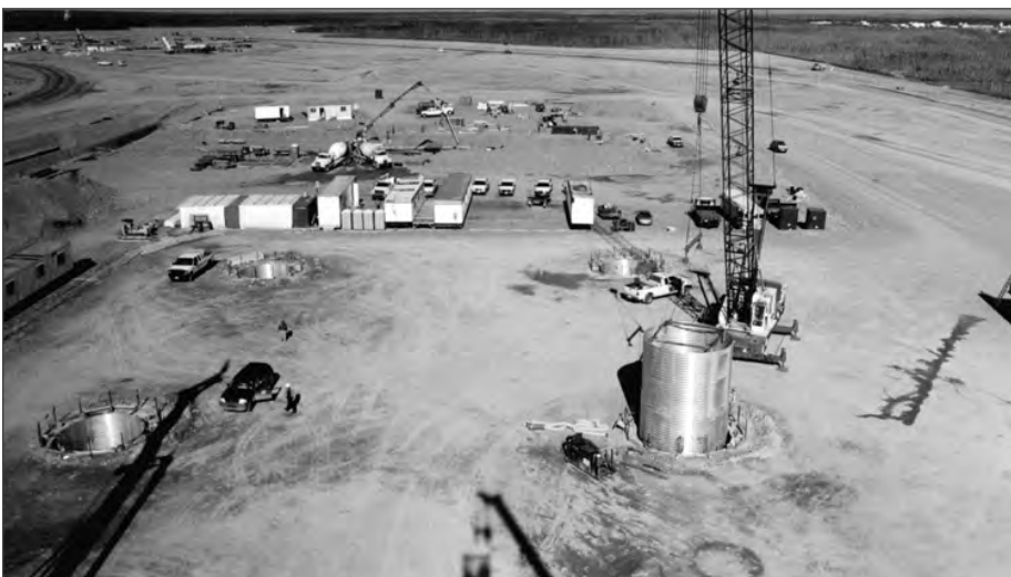
■ Inserting the structural plate shaft liner.
