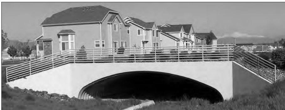
■ Housing Development in Thornton, Colorado. Super Cor Box Culvert 35'-9" span x 7'-9" rise.
