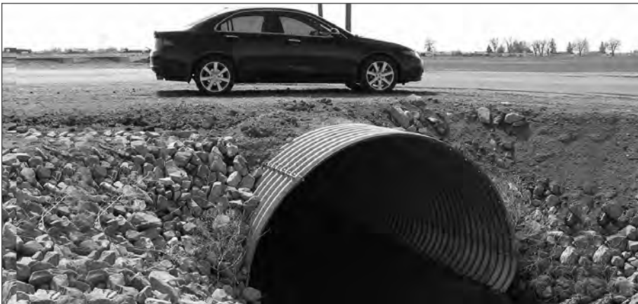
■ Structural plate pipe arch for an irrigation ditch crossing.
