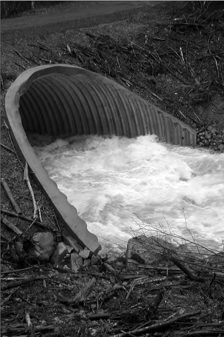
■ Deep corrugated structural arch during high flow.
