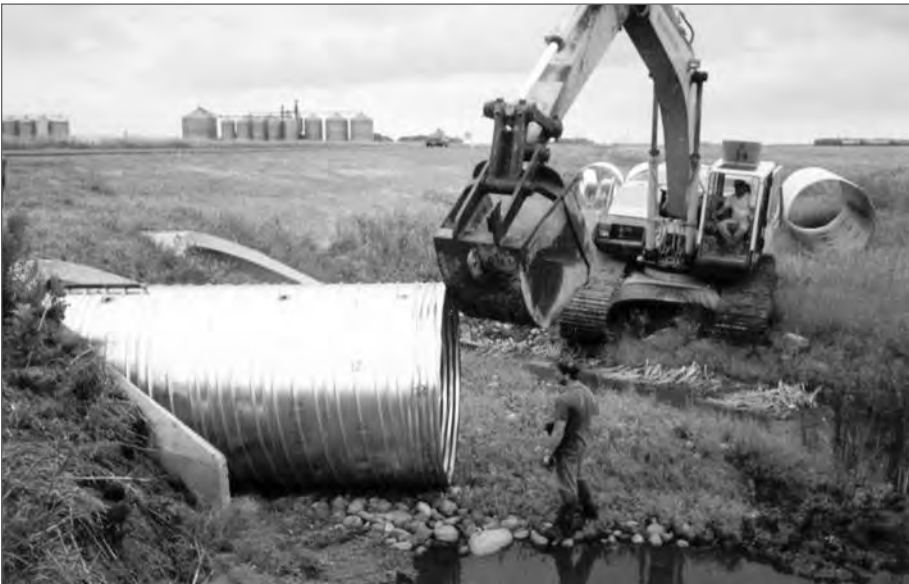
■ Figure 12.5 Liner pipe is easily installed by pushing or pulling through host pipe using conventional equipment.
