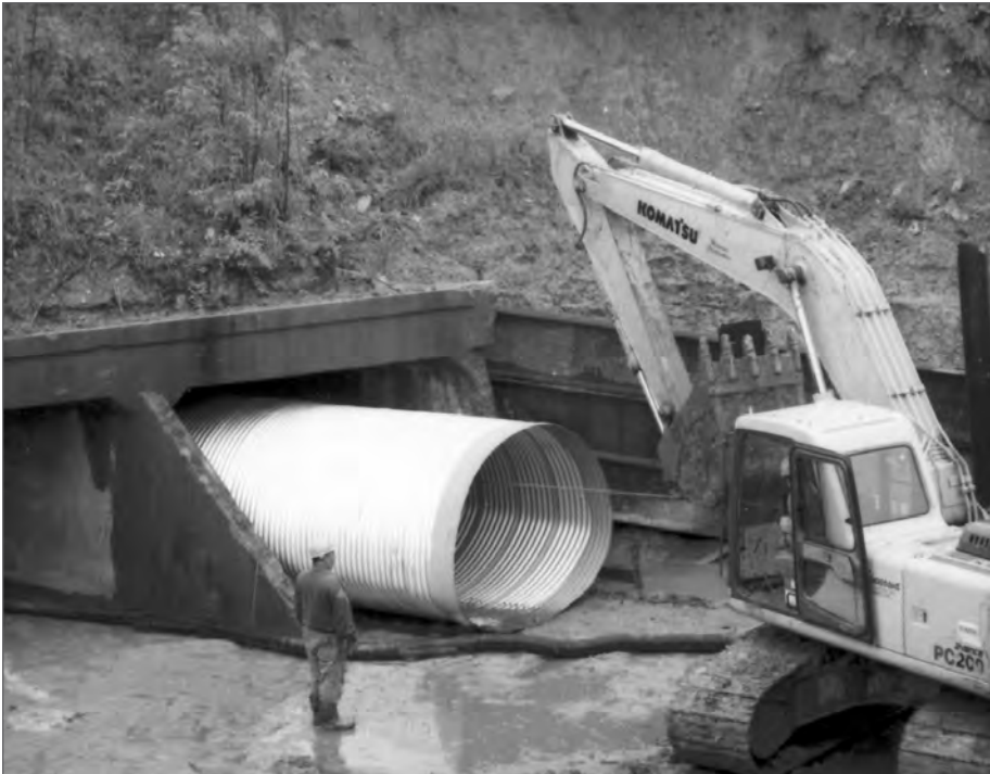
■ Figure 12.6 Liner pipe being installed in an existing concrete box.
