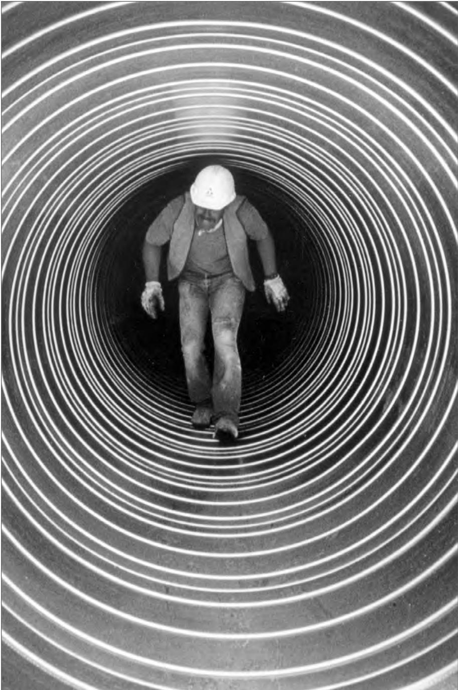
■ Figure 12.1 Pipe inspection.
