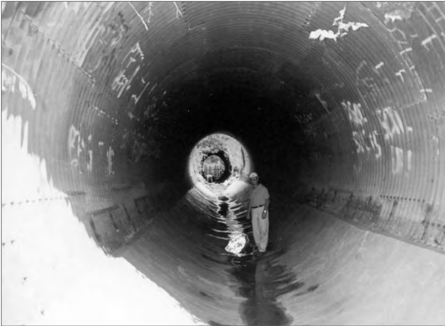
■ Figure 12.18 Concrete paved invert in structural plate pipe.
