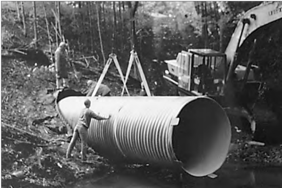
■ Figure 12.19 Slip lining with CSP.
