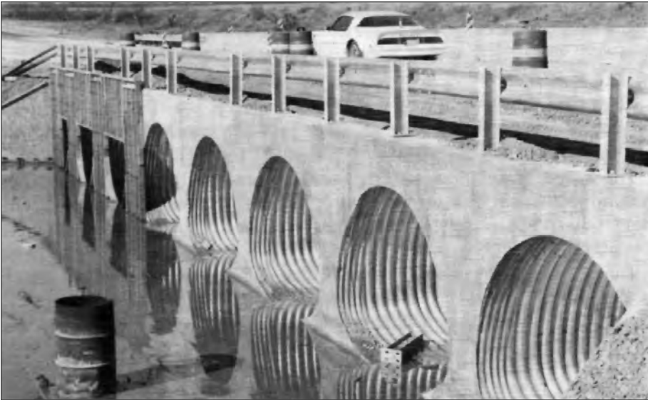
■ Figure 11.4 Texas DOT bridge replacement project. After...
