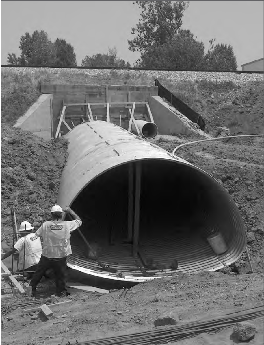
■ Rehabilitation & extended concrete box.
