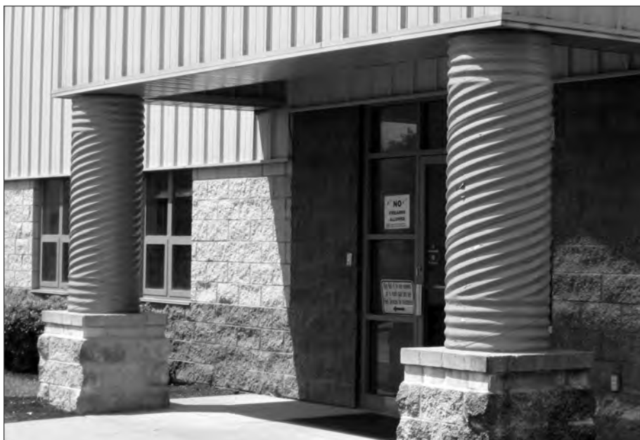
■ CSP entry columns for commercial building.
