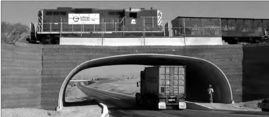
■ Structural plate grade separation between railroad and highway.
