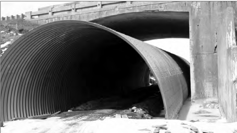
■ CSP bridge replacement provides an economical installation with short road closure time.
