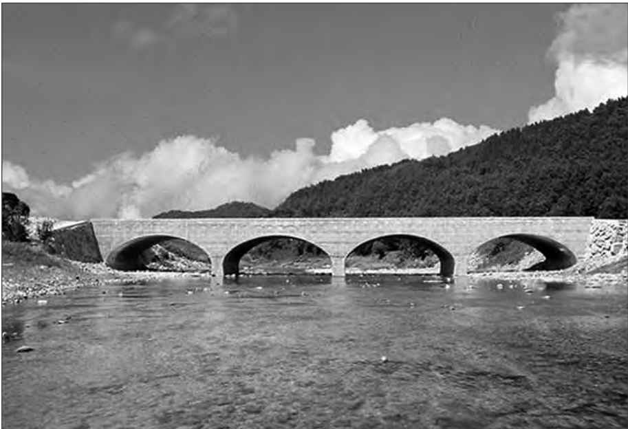
■ Corrugated steel structural plate bridge structure.
