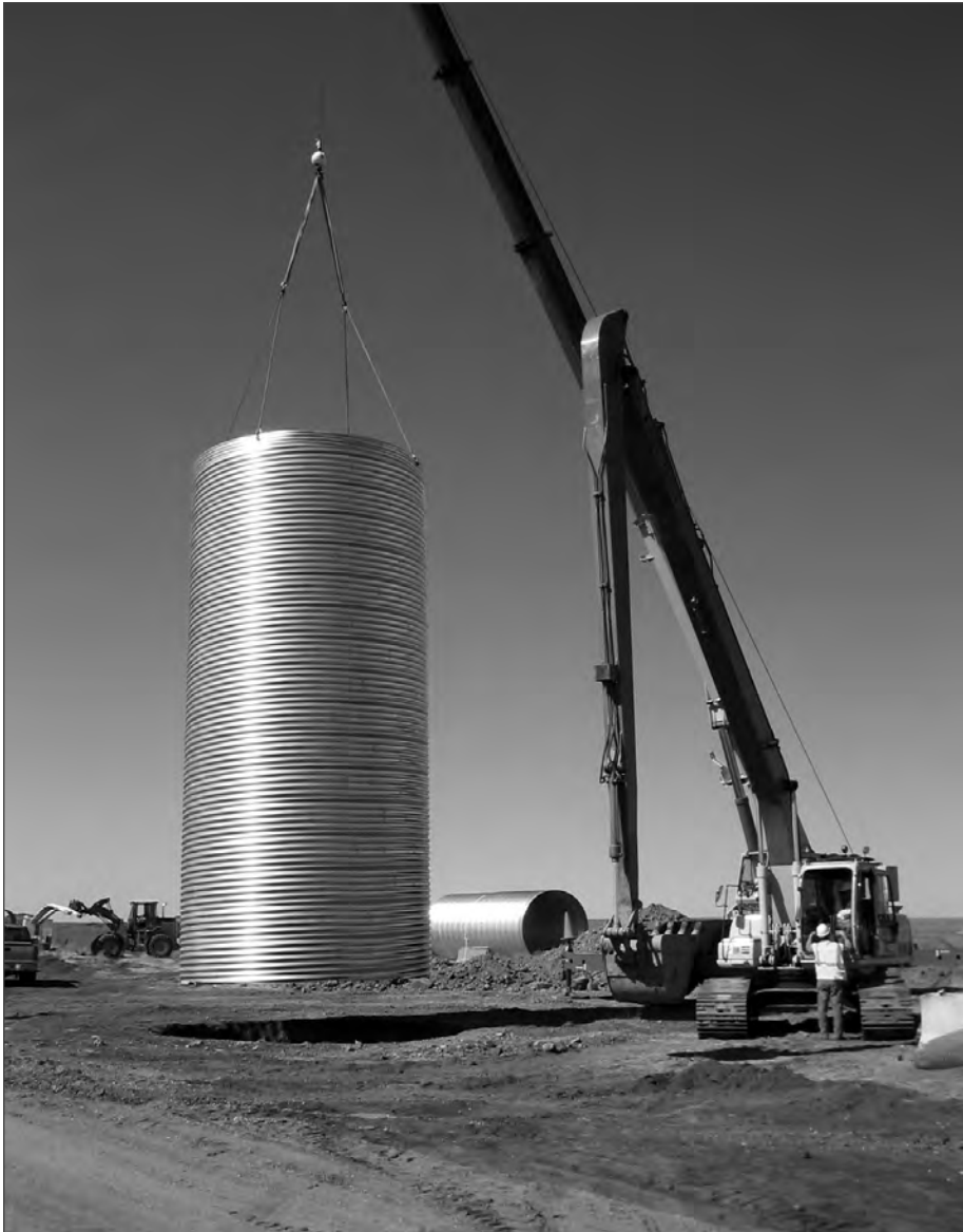
■ CSP form for wind turbine generator footing.
