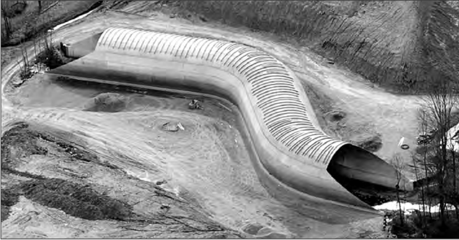
■ Structural plate structure following curvature of a natural stream.
