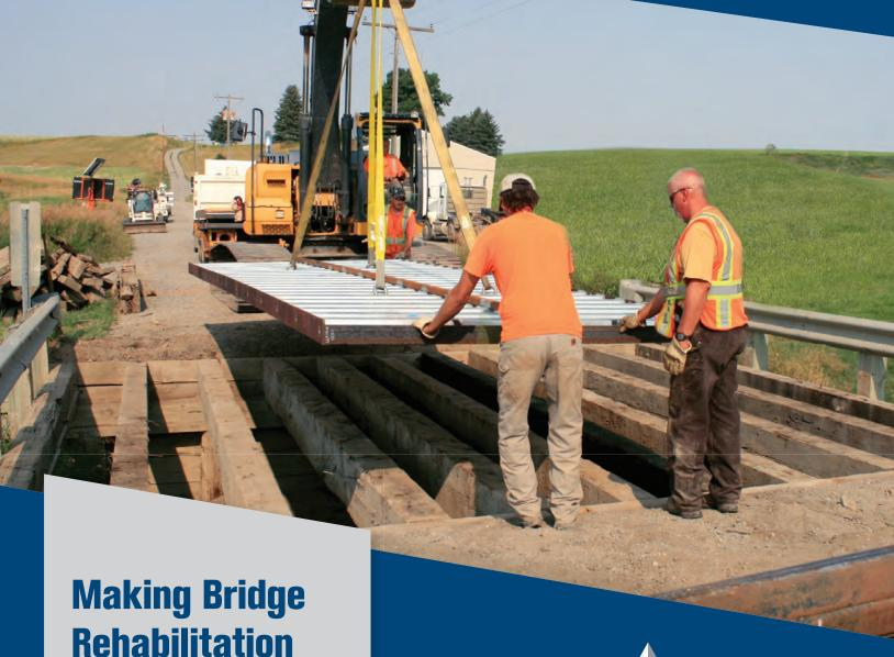
TrueNorth Steel's innovative process uses lightweight prefabricated galvanized corrugated steel deck panels. RediDek™ bridge deck panels arrive on site ready to install on existing steel, wood or concrete girders.
