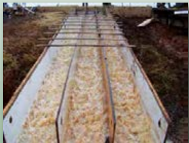
Medium Flow In Channel
