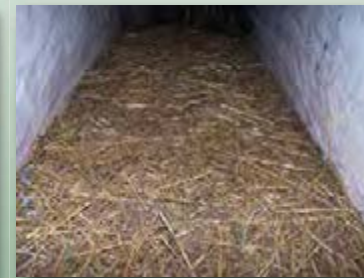
Channel After Matting Removed (no apparent soil surface disruption)
