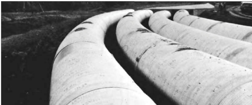
■ Moderate horizontal curvature in a culvert or sewer can be achieved with ordinary couplings. Greater changes in alignment will require fabricated fittings.
