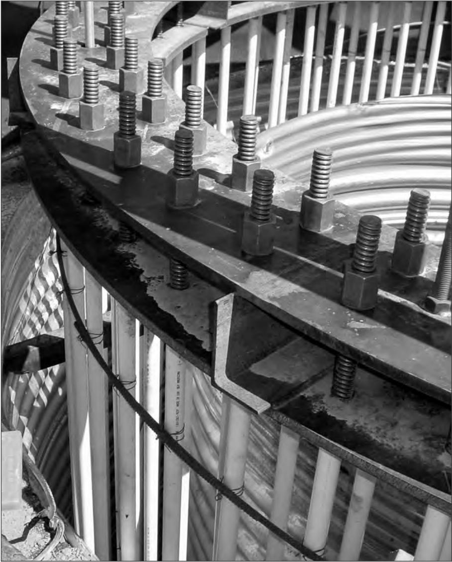
■ CSP form for wind turbine generator footing.
