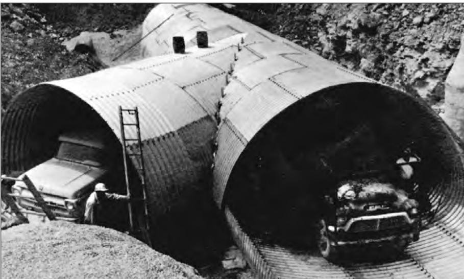
■ King-size wye or lateral for large storm sewer was shop-assembled, then dismantled and shipped to the job site for final erection.
