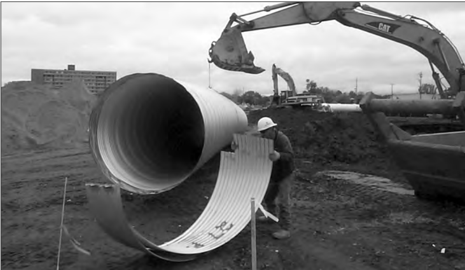
■ Two-piece bands being installed on reformed ends of CSP.
