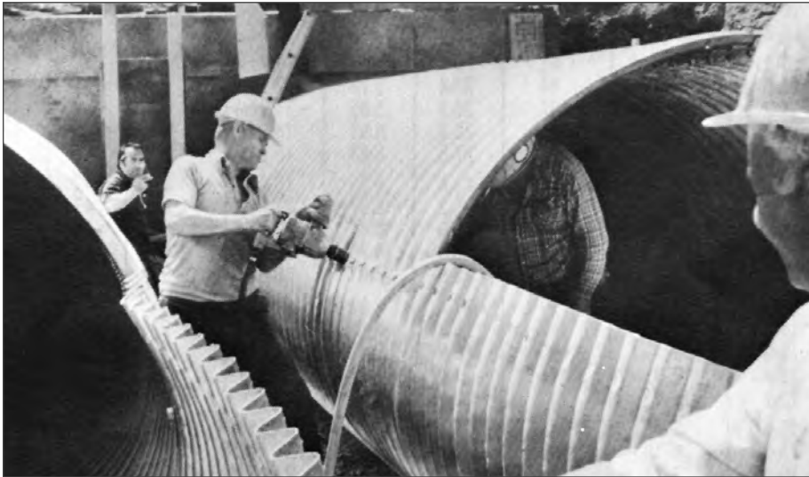
■ Figure 2.9 High-strength steel bolts are used for the circumferential and longitudinal seams of structural plate pipe. Four, six, or eight bolts per foot of longitudinal seam provide the strength required for the loading conditions.
