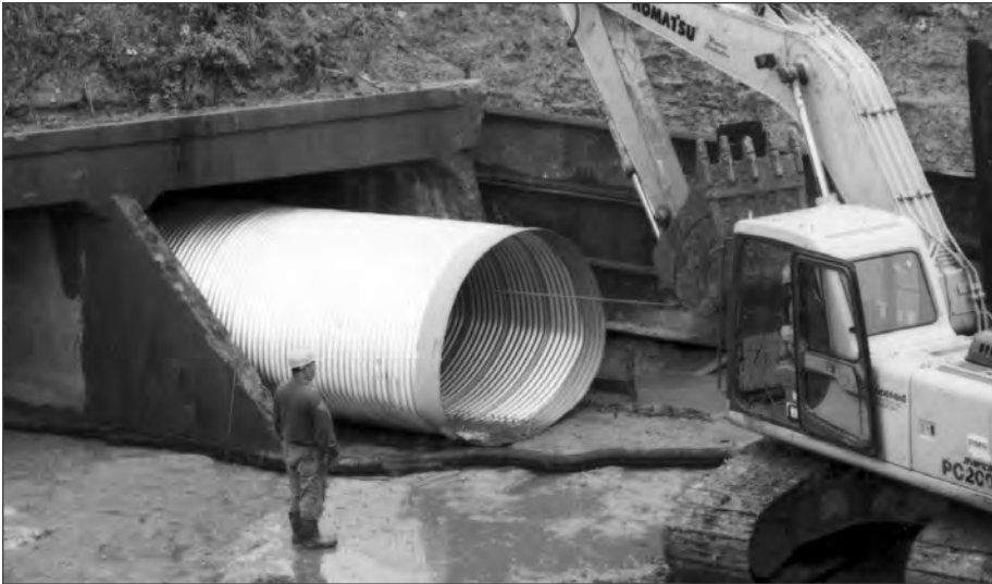
■ Relining of a failed concrete box with corrugated steel pipe arch.
