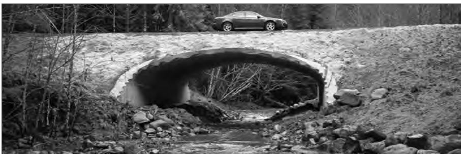
■ 36 foot span by 10 foot 5 inch rise deep corrugated box culvert with beveled ends, used for a Fish Passage project in the Willamette National Forest in Oregon.
