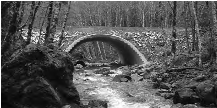
■ 35 foot span by 15 foot rise deep corrugated structural plate arch with beveled ends for a Fish Passage Project in the Willamette National Forest in Oregon.
