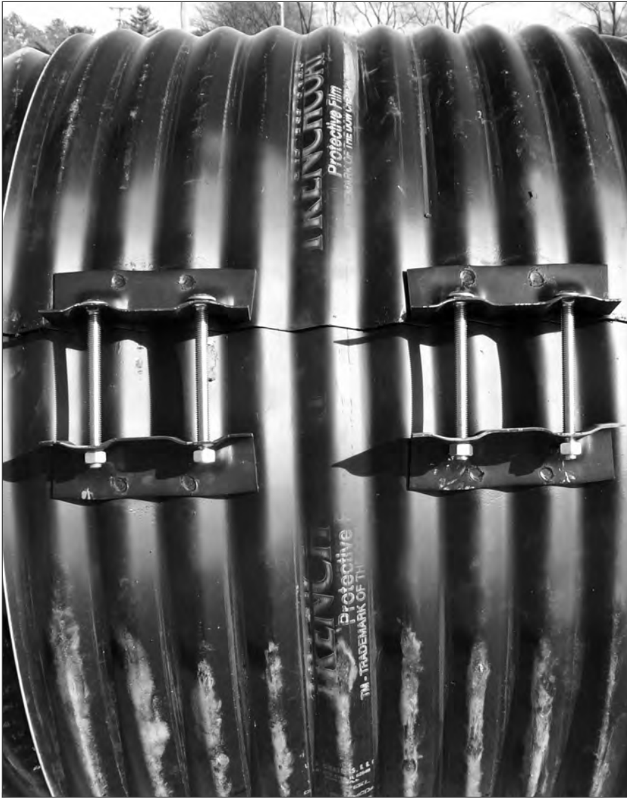
■ Corrugated steel pipe band connectors.
