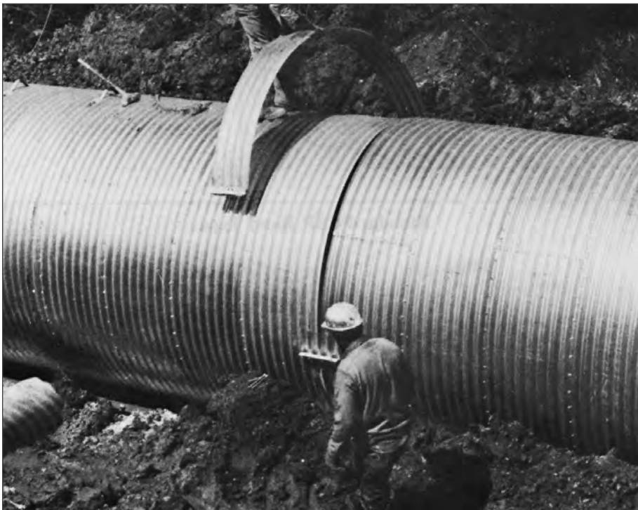
■ Two-piece corrugated band joins length of annular riveted pipe.
