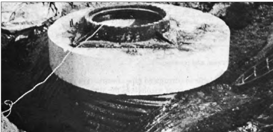
■ Standard cast iron covers and/or steel grates are used with CSP manholes and catch basins.
