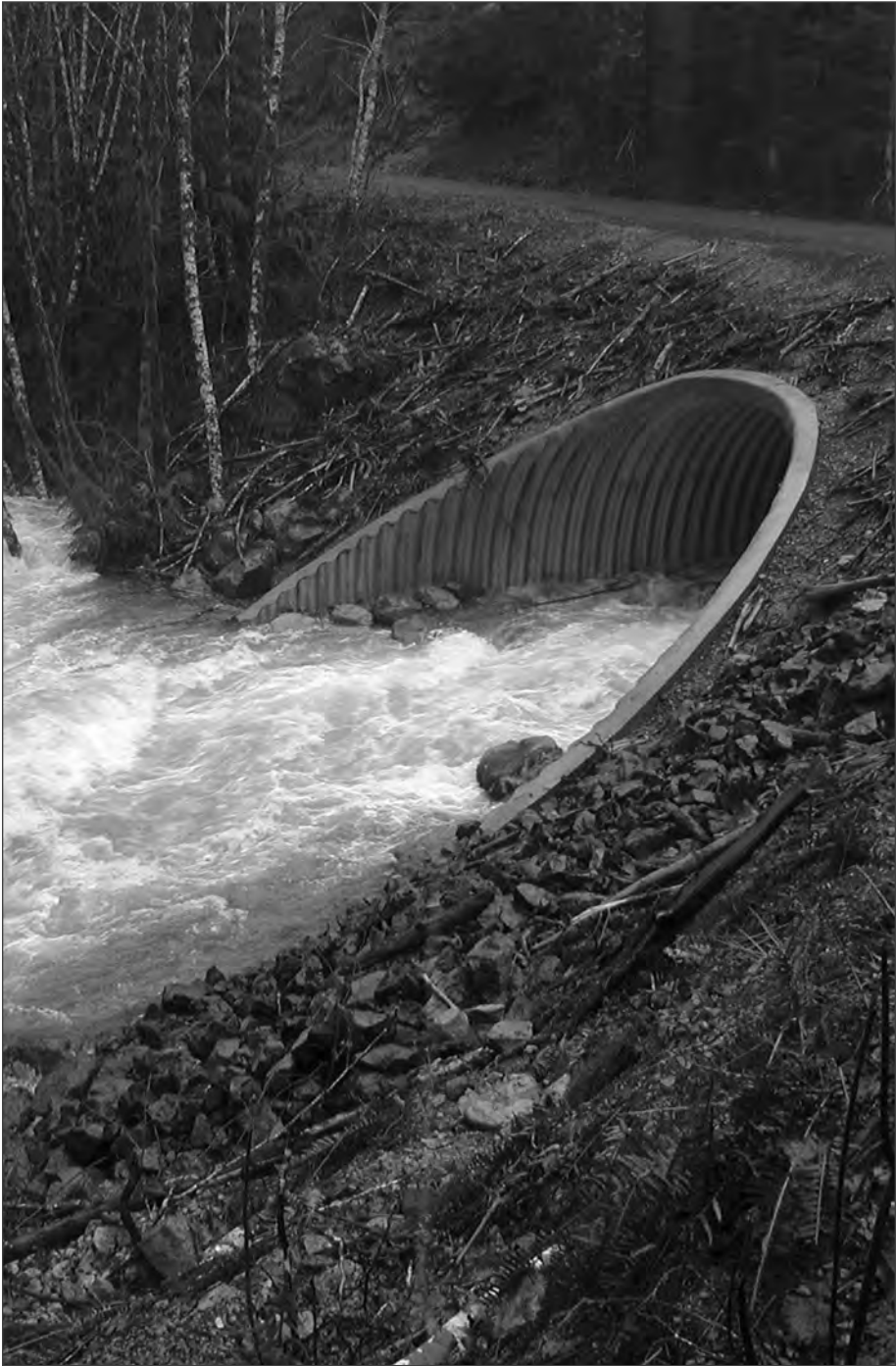
■ Deep corrugated structural plate arch during high flow.
