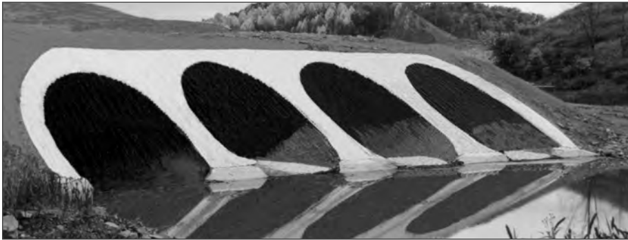
■ Figure 10.31 Multiple line CSP beveled ends.
