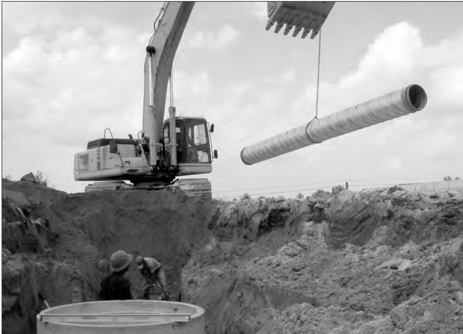
■ Figure 10.12 Lifting CSP into place.
