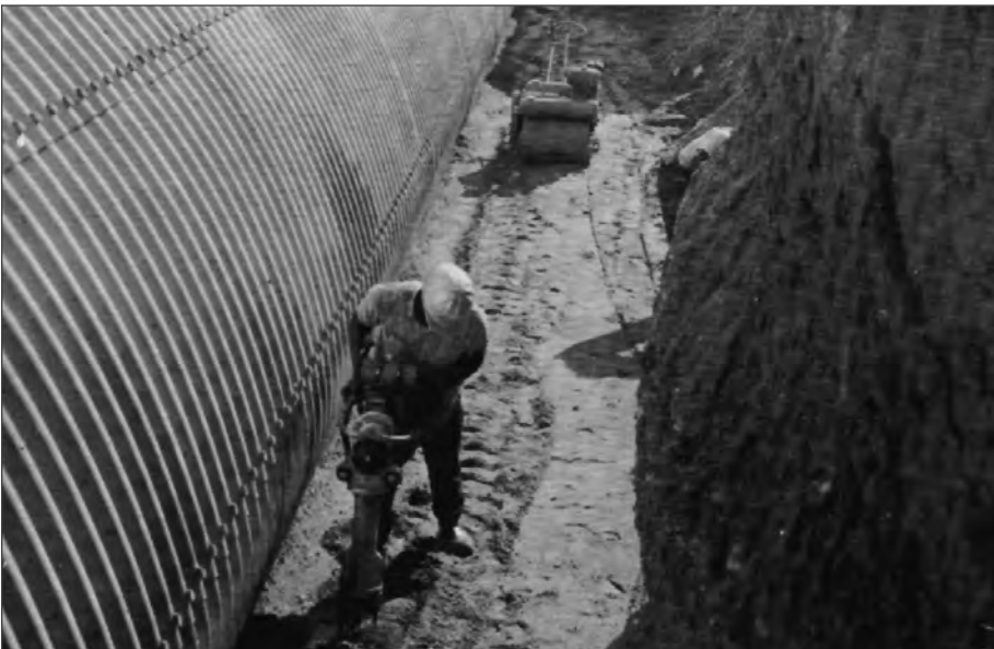
■ Figure 10.22 Proper use of Compaction Equipment.
