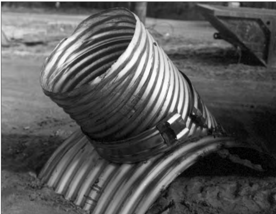
■ Figure 10.18 Typical CSP saddle fitting.
