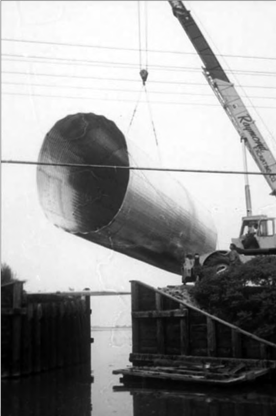
■ Figure 10.44 Assembled structure being placed in position.
