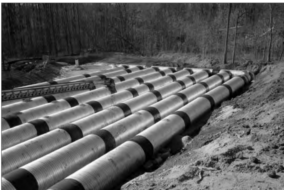
■ Figure 10.13 CSP pipe joints wrapped with geosynthetic wrap.
