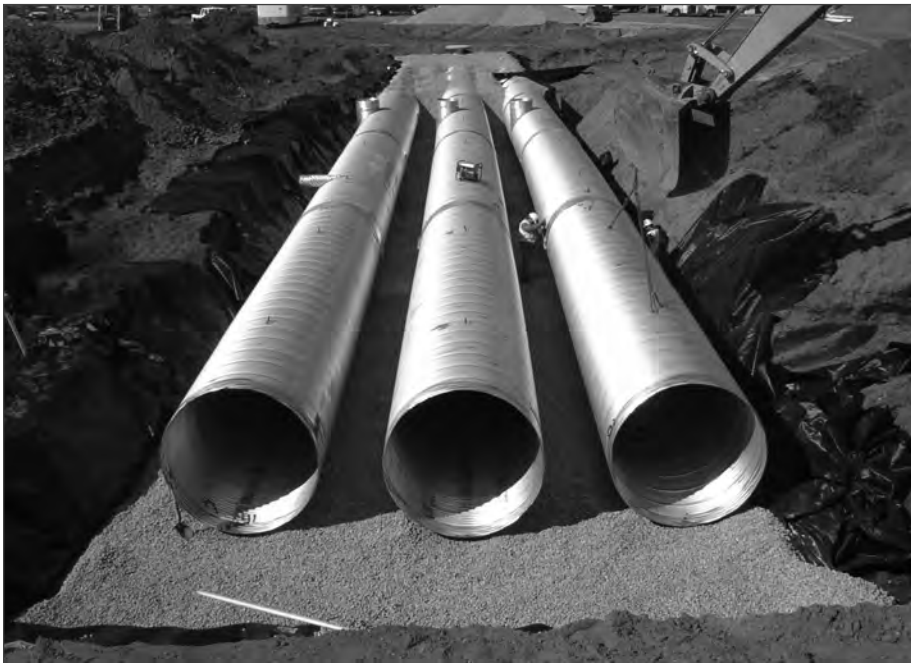
■ Figure 10.33 Detention system installation.
