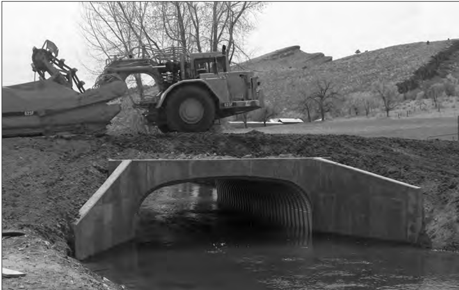
■ Box culvert with construction equipment loading on top of the structure.
