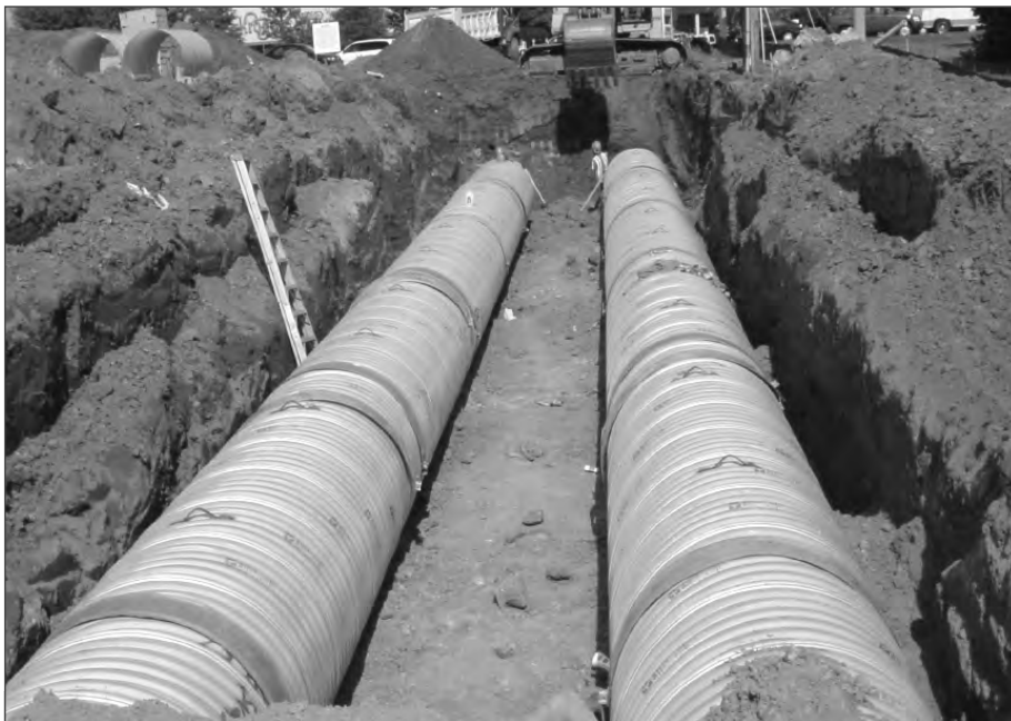
■ Figure 10.8 Proper bedding is important for multiple barrel installations.
