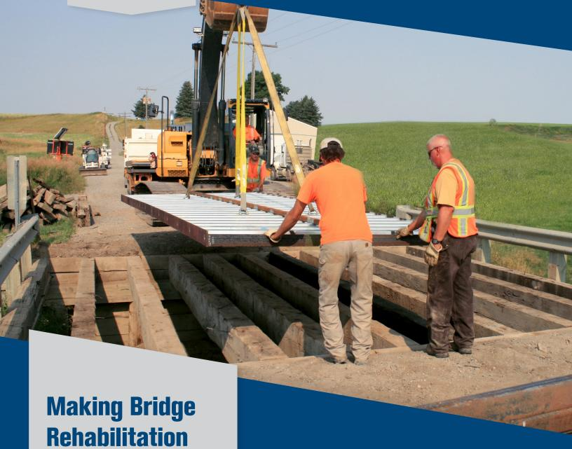
TrueNorth Steel's innovative process uses lightweight prefabricated galvanized corrugated steel deck panels. RediDek® bridge deck panels arrive on site ready to install on existing steel, wood or concrete airders.
