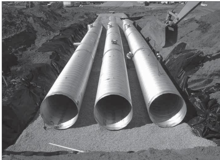
■ Figure 10.33 Detention system installation.
