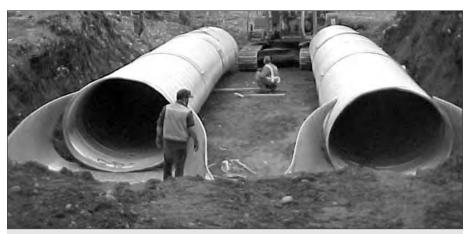
**Figure 7.24** Pipe arch can be installed in limited headroom situations with shallow cover.
